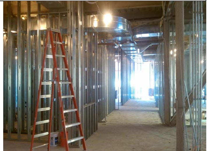
First Floor Framing & Rough OH Mechanical
