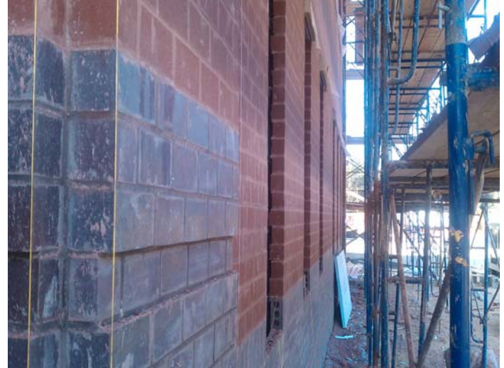
Brick / Rigid Insulation – East Elevation
