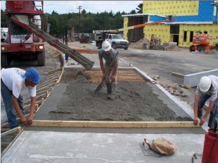
Infiltration Bed #2 Installation (Phase II Scope – Ahead of Schedule)
