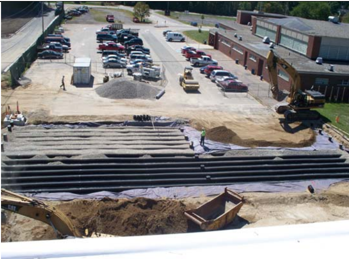
Infiltration Bed #2 Installation (Phase II Scope – Ahead of Schedule)
