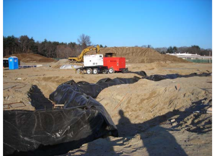
West Wall Weather Protection Blankets & Heat
