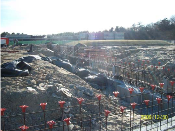
Forming Walls @ W Side of Bldg
