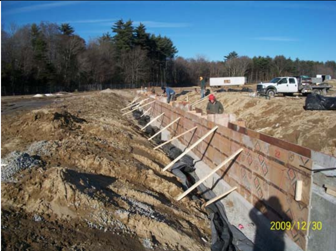
Forming Walls @ W Side of Bldg
