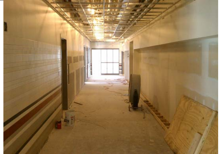
2 nd Floor Ceiling Grid and OH MEP Rough
