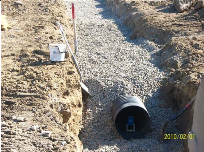
Underslab Electrical Conduit Installation
