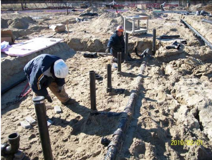
Drainage Installation @ South Parking Area
