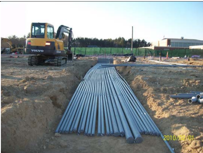
Underslab Electrical Conduit Installation
