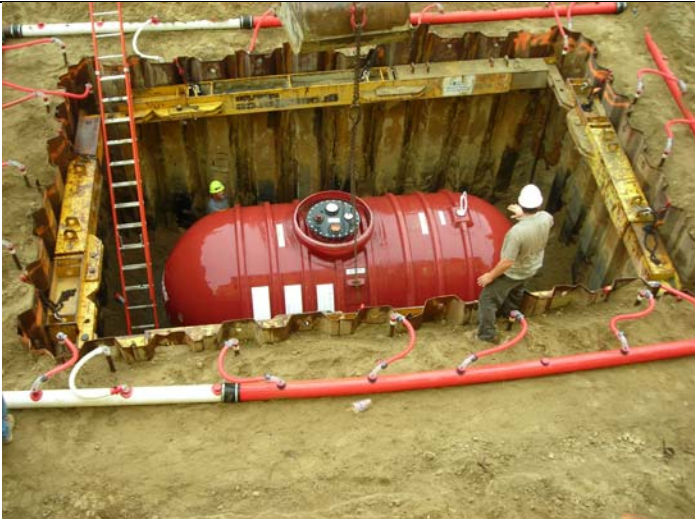
Tight Tank Installation
