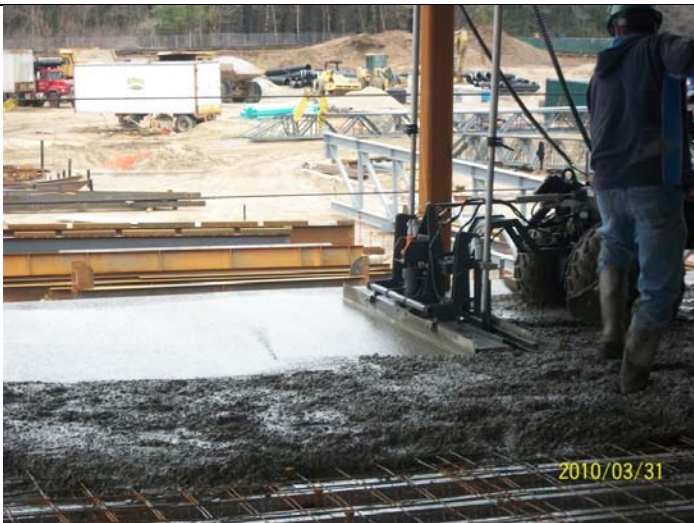
2 nd Floor Concrete Slab on Deck Placement
