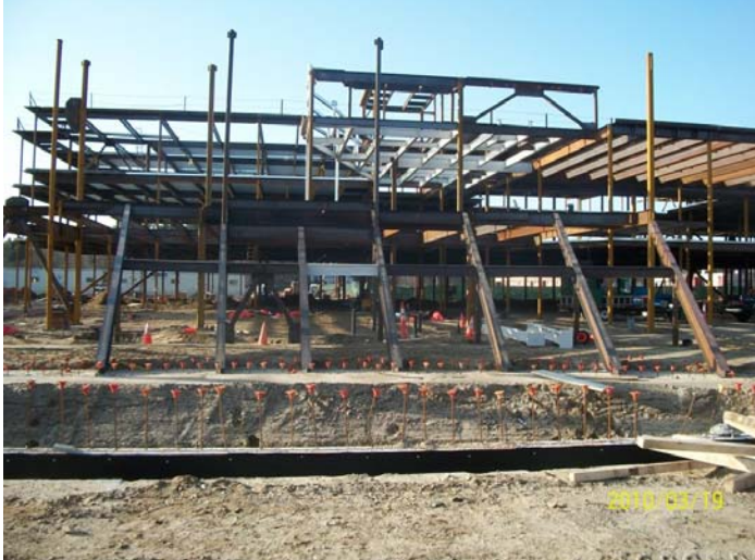
2 nd Floor Steel Decking & Wire Mesh
