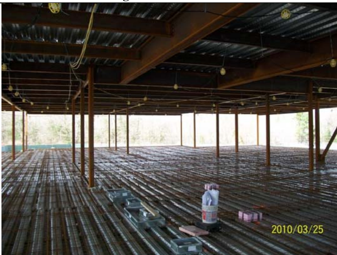
2 nd Floor Concrete Slab on Deck Placement
