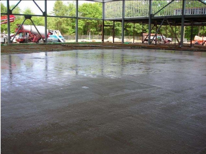
Gymnasium Slab on Grade Placement
