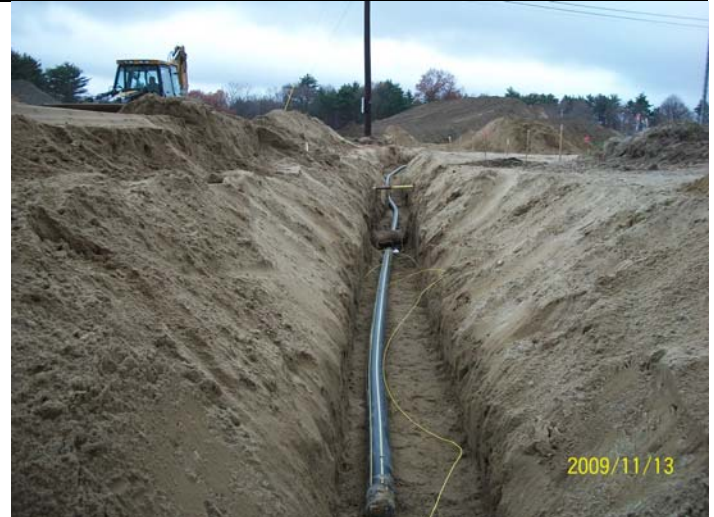
New Gas Line Installation
