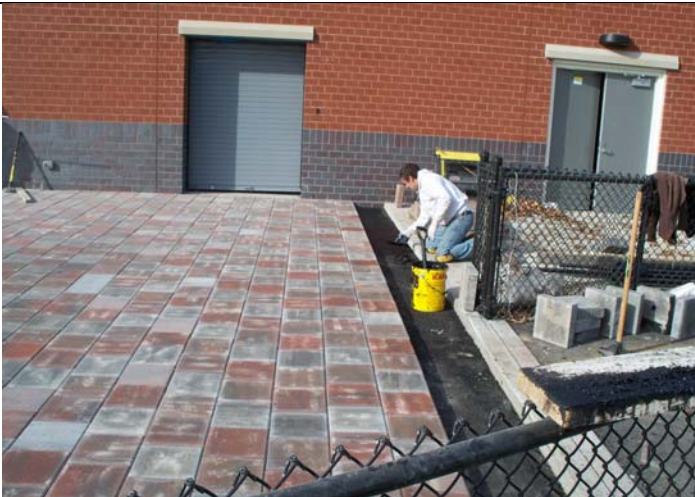
Concrete Unit Pavers @ Concession Stand
