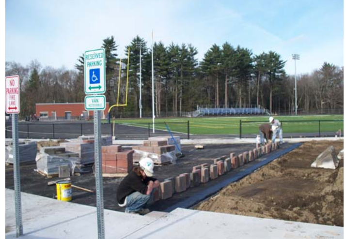
Concrete Unit Pavers @ Maintenance Bldg
