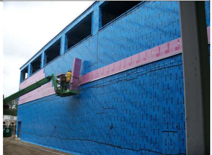
Insulation / Prep for Metal Wall Panels
