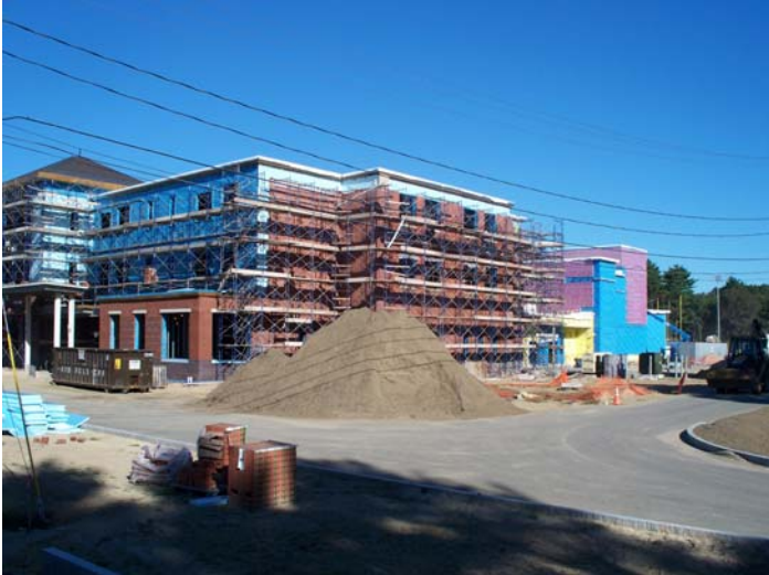
Temp Weather Protection Installation
